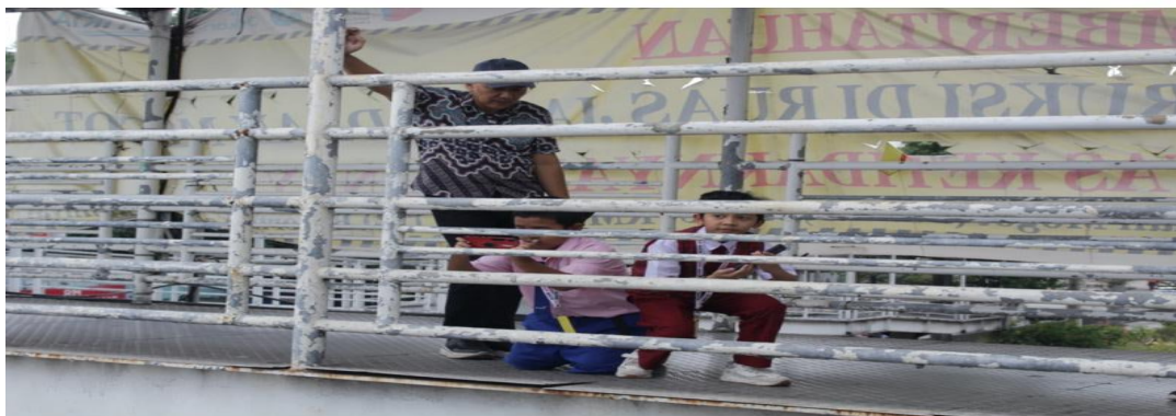
Safe elevated pedestrian bridge (JPO) views] .
