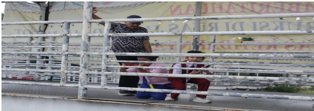
Safe elevated pedestrian bridge (JPO) views] .
